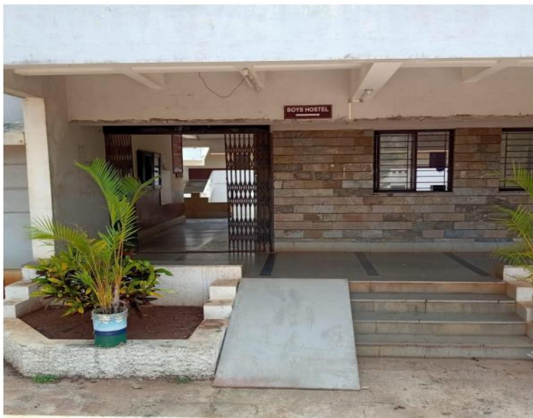
Hostel & Mess Ramp Facility
